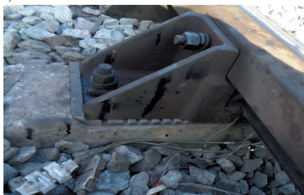
Fig. 3. Turnout switch type P65, grade 1/11, equipped with experimental rail pads* * Photo made by the author
